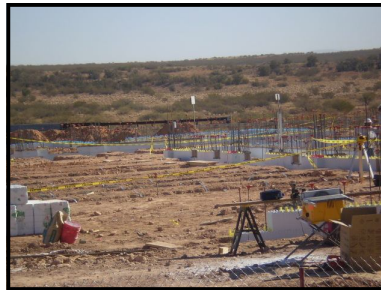
Construction continues at the site. / Continua la Construcción
